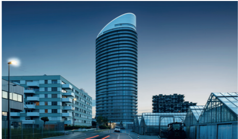
Jabee Tower Dübendorf
