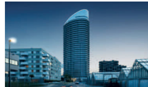
Jabee Tower Dübendorf
